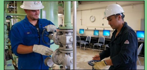
Two students are hard at work on Process Operating equipment
