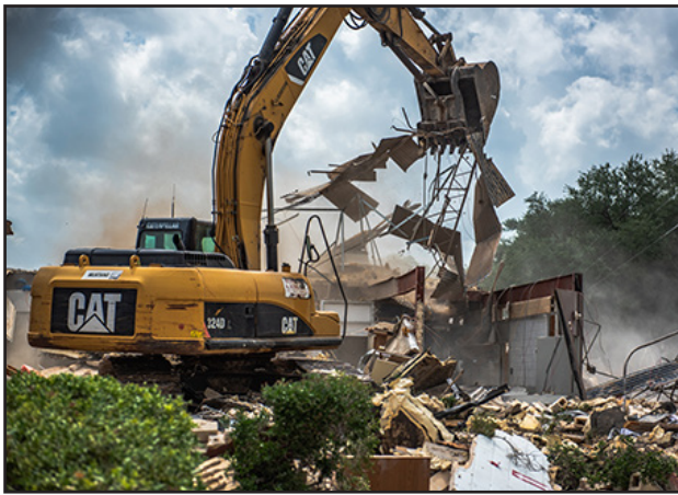
Demolition of the T1 building begins.
