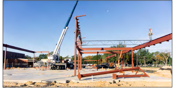
Construction workers install the frame on the new Student Services Building.
